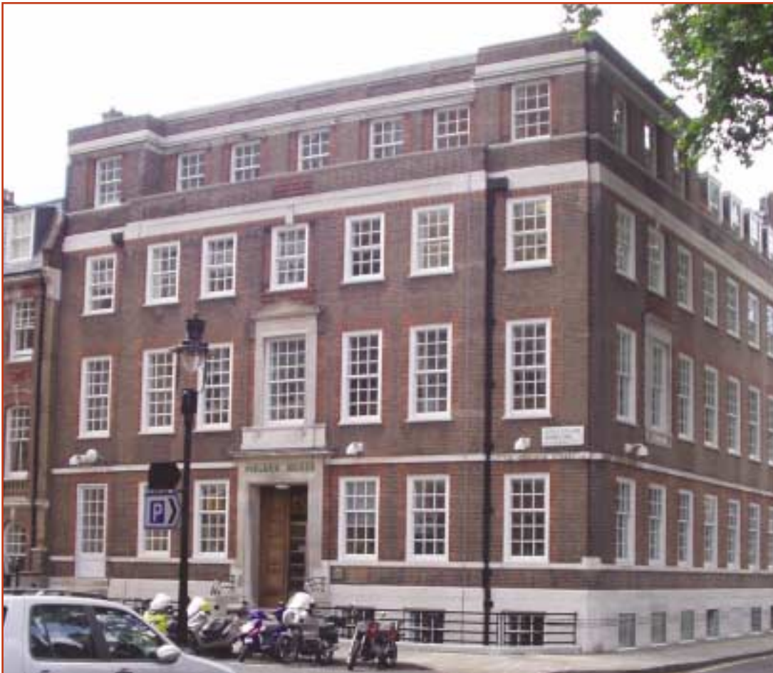
Fielden House, occupied in January 2005, provides accommodation for Members and their staff as well as three meeting rooms.
